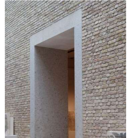
Concrete Lintels, surrounds and cills – Painted White
